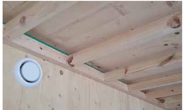
DOUBLE SEPARATION FOR A SUSPENDED CEILING
